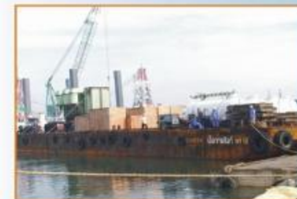
Phu My 3 Power Station with transformer 220tons from Singapore to erection position, Phumy Vietnam, Jan-2008
